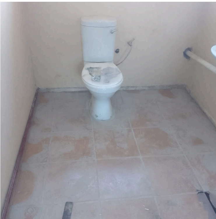
Ablution facility completely revamped with new tiles installed.
