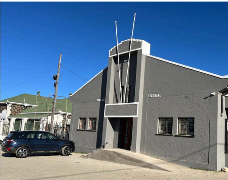
The building received a fresh coat of paint with a new staircase and ramp.
